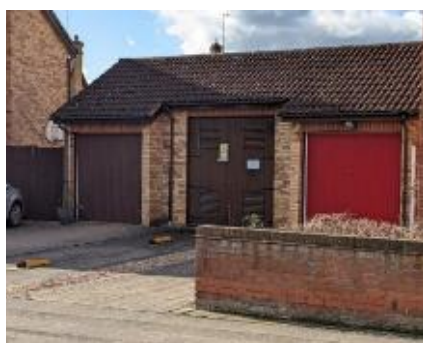
Baron Court: Disguised sub station
