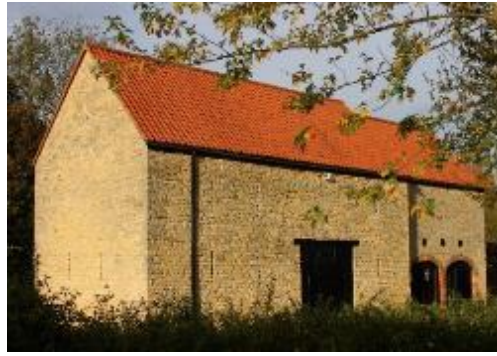
Former Outbuildings of Fox Covert Farm, now The Barn Youth Centre
