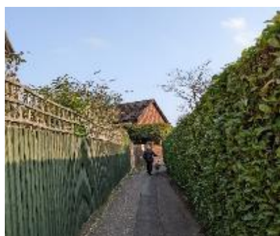
Lakeside: hidden substation
