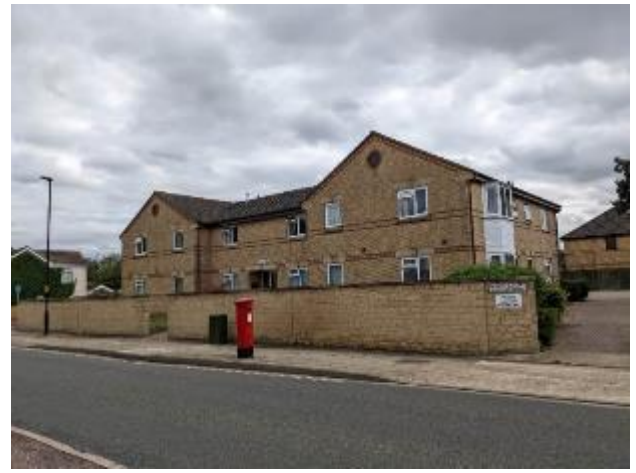
Poor development, Wren Court
