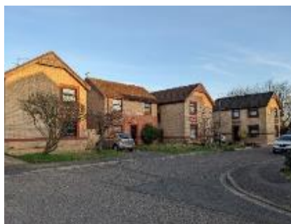
Hazelcroft: Decorative brickwork
